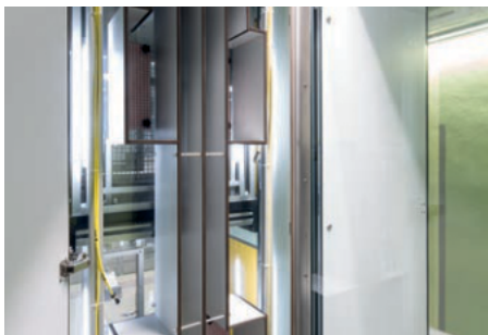
Fig. individual interior equipment
