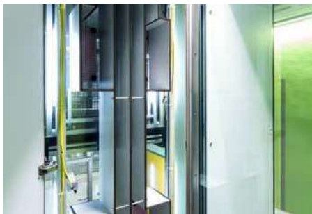
Fig. individual interior equipment
